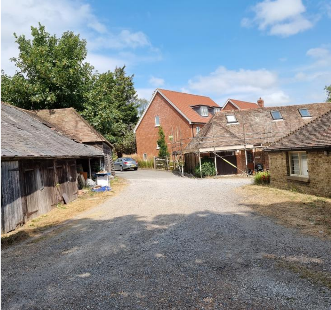
Fig 7. Cart store & Granary to left of photo. Other curtilage listed buildings within Ingles Yard to right of photo with new housing development in background. (Former Garden Centre site). Trees in the background to remain with a new hedgerow to be planted facing the west boundary, as set out on page 23 of the DAS.
