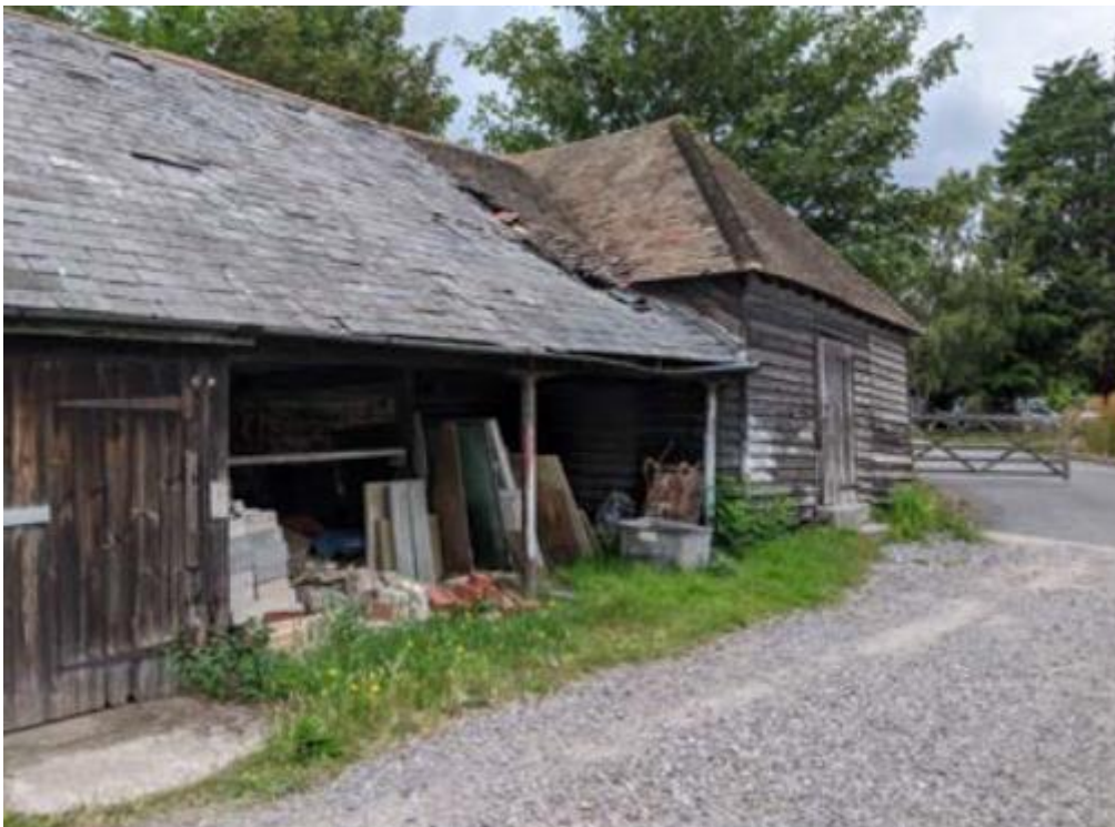
Fig.3 Front (west) elevation. Cart store (in foreground) with Granary building
